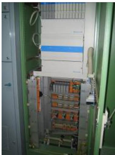
Coating line is equipped with Honeywell drive control system TDC
